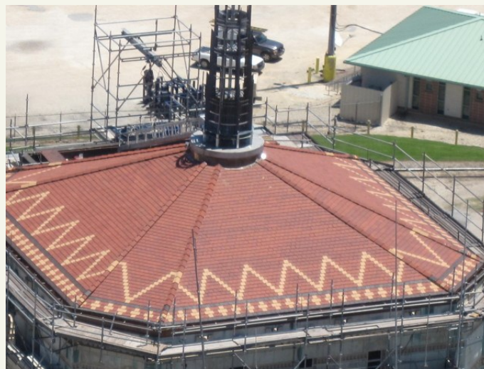
1931 Jefferson County Courthouse Roof— a rarely seen aerial view from 2009 repairs.
